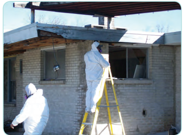
Preparation for Asbestos Abatement
