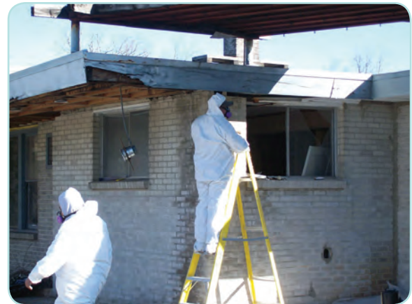
Preparation for Asbestos Abatement
