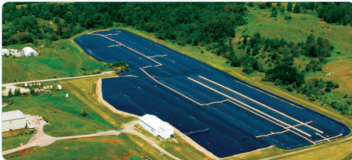
Aerial View of State Disposal Area
