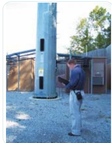
Christopher Green conducting a recent site inspection of a collocation cellular tower site.
