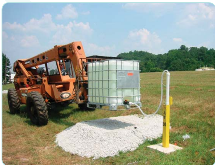
Figure 3. Installation of Injection System
