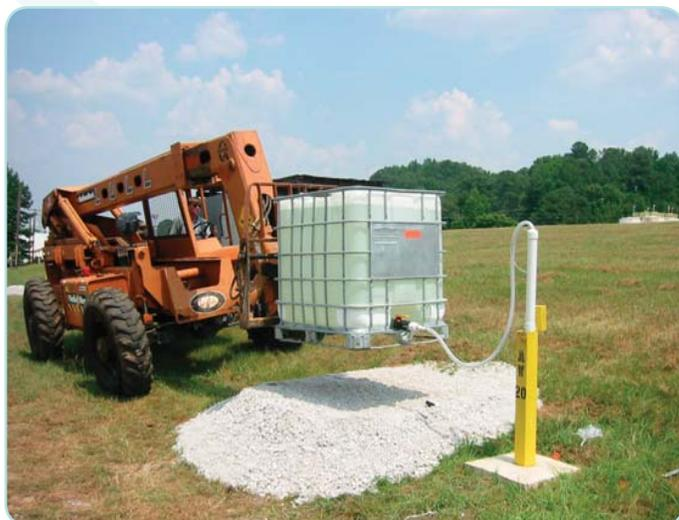
Figure 3. Installation of Injection System
