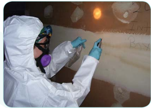
Asbestos Sampling
